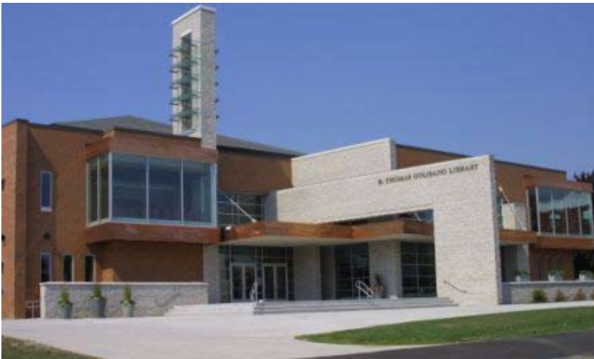
The B. Thomas Golisano Library at Northeastern Seminary uses a geothermal HVAC system.
