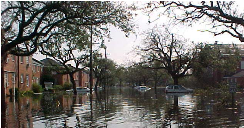
Student and staff housing (left) sustained extensive damage from the flood waters that filled DeMent Street (named after NOBTS's first president). Buildings to the right, including the chapel, sustained wind damage, resulting in water leaks through the roofs.
